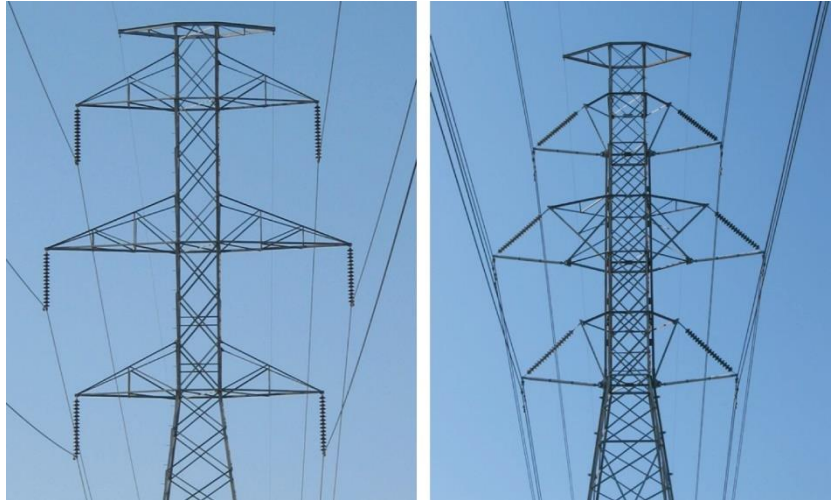
Figure 6-67 230-kV structure prior to conversion to 345 kV [1]
