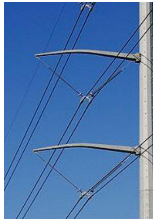
Figure 6-89 Aesthetically pleasing lines on gull-wing cross-arms
